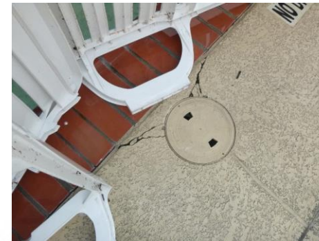
Deck/skimmer cracking
