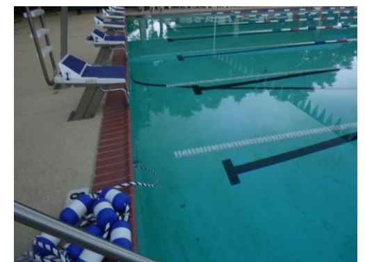
Figure 1.2, Area of large crack
