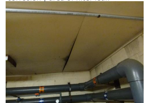
Figure 1.42 Mechanical room ceiling damage
