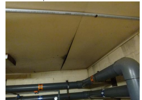
Figure 1.36, Mechanical room ceiling damage
