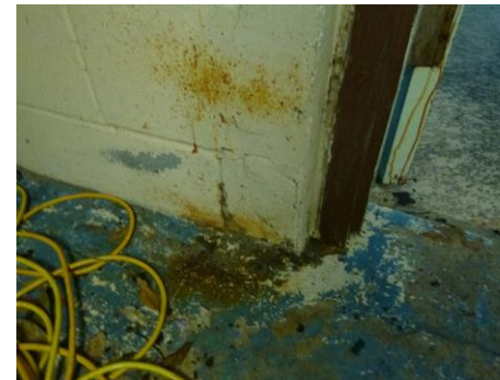
Figure 1.41, Wall/door deterioration
