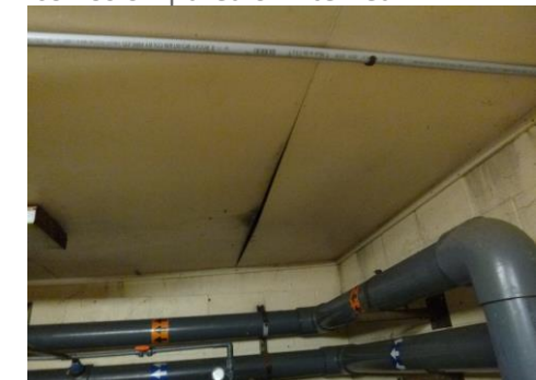
Figure 1.30, Mechanical room ceiling damage
