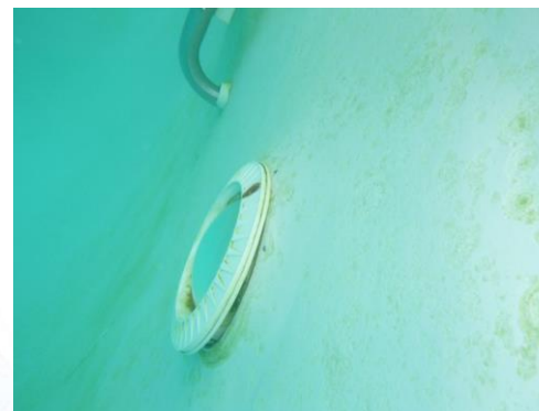
Figure 1.5, Underwater light not in place
