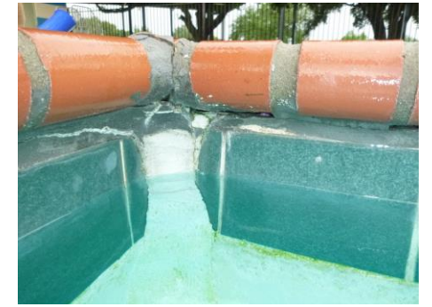
Figure 1.7, Coping stone loose and cracking
