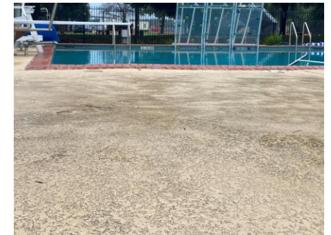
Figure 1.12, Uneven/shifting concrete deck and pool
