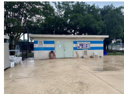
Figure 1.23, Pool mechanical building
