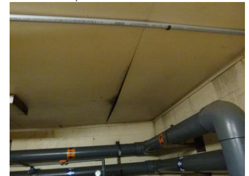
Figure 1.36, Mechanical room ceiling damage
