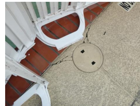
Deck/skimmer cracking
