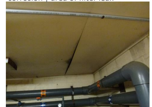
Figure 1.42 Mechanical room ceiling damage
