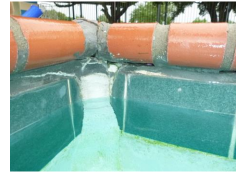
Figure 1.8, Area of corner wall repair
